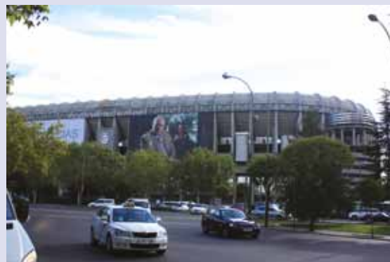
The Bernabéu Stadium
